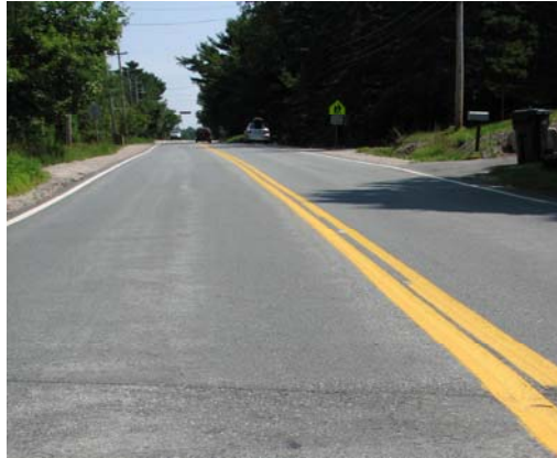
Passing lane eliminated in front of school—dashed line painted over
